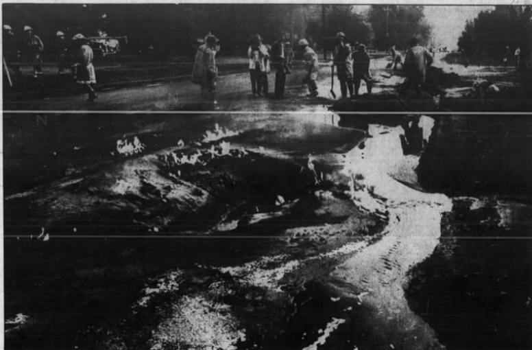
The break in the pipeline caused this hole in the pavement on Long Lake Rd. in Mounds View. Firefighters used sand to contain the fire.
